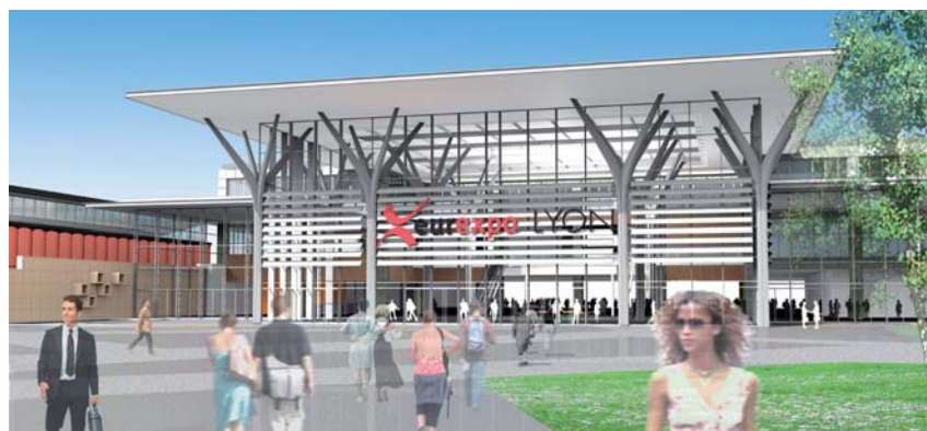
The new Welcome Area of Eurexpo Lyon is to be opened in September 2010.
